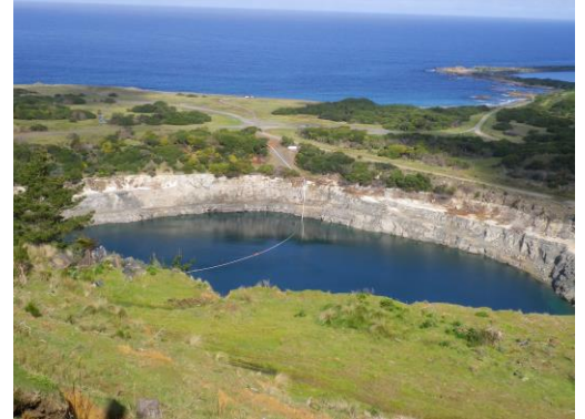
Dolphin open cut mine undergoing dewatering- Aug 2014
