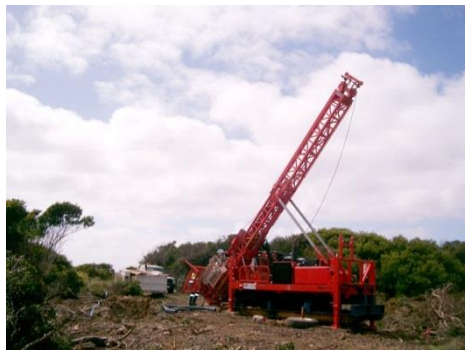
Drilling rig conducting geotechnical work
