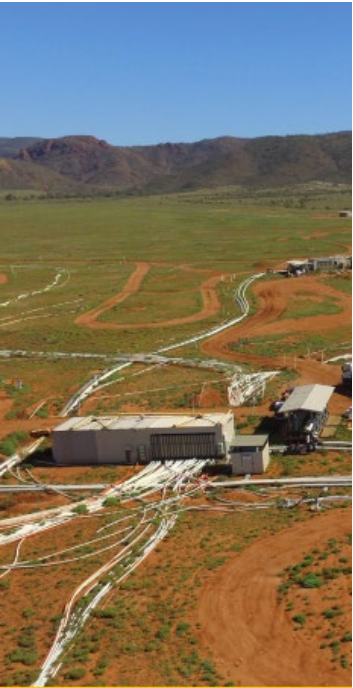
Aerial view of Four Mile uranium well house. (Courtesy Heathgate Resources; photo 415063)
