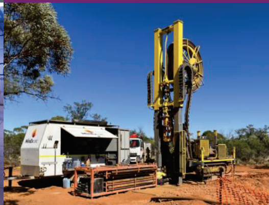
Coil tube drilling rig
