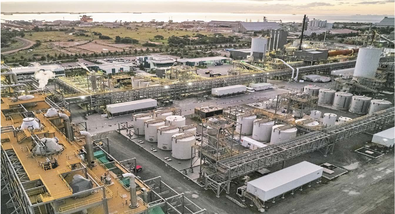
Tianqi's Kwinana lithium hydroxide plant. CREDIT: Image courtesy of Tianqi.
