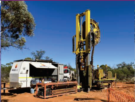
Coil tube drilling rig
