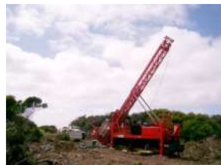
Drilling rig conducting geotechnical work
