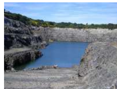
Dolphin open cut mine, dewatering underway
