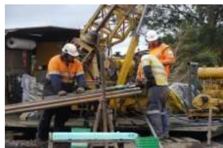
Drilling rig at Heemskirk
